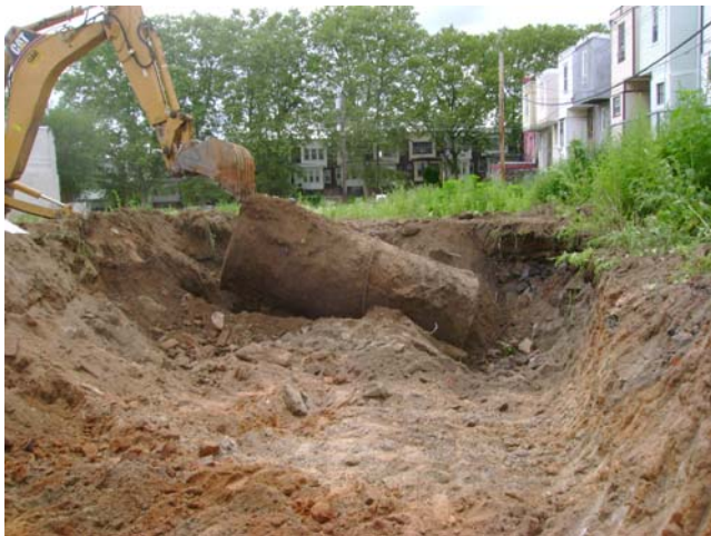
Storage Tank Closure
