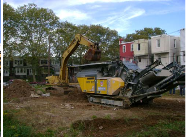
Materials / Debris Crushing
