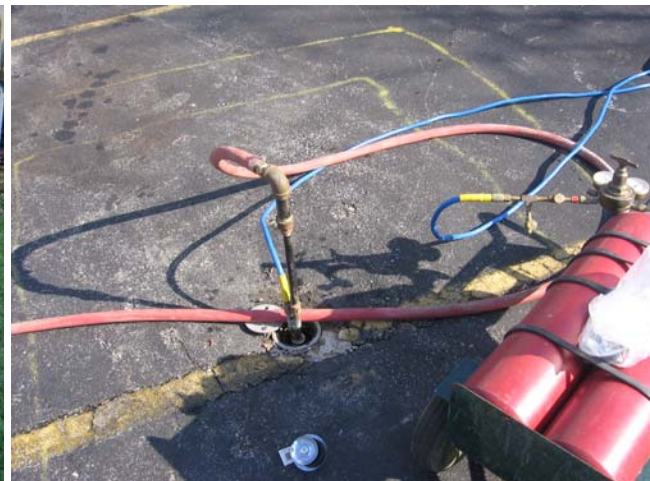
Microbe and Nutrient Injection
