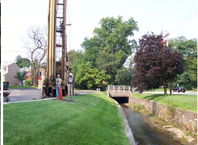
Injector Point Installation
