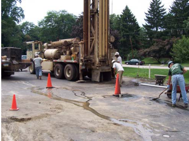
Injector Point Installation
