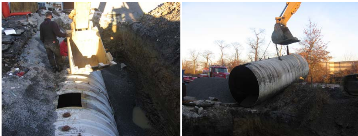
Storage Tank Excavation
