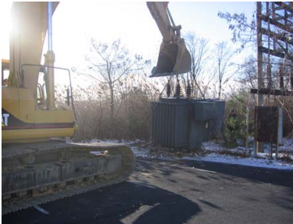
Transformer Removal
