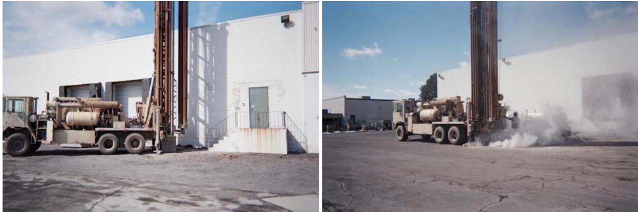
Monitoring Well Installation (Air Rotary Drilling Method)
